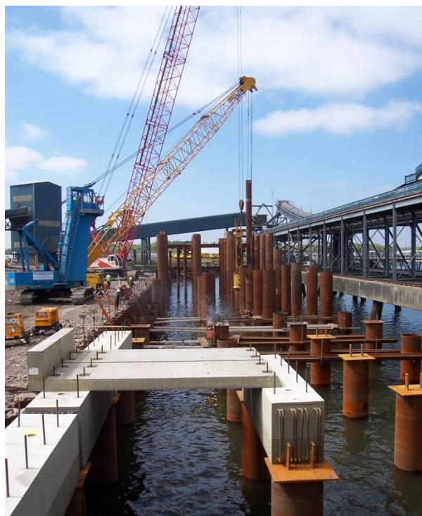
Figure 11: Photograph illustrating typical Quay Construction.
