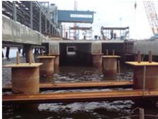
Figure 11: Photograph illustrating typical Quay Construction.
