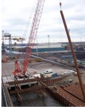
Figure 6: Photograph illustrating a Steel Tubular Pile being 'Pitched'
