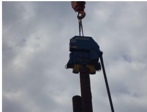
Figure 7: Photograph illustrating a Vibro Hammer driving a Steel Tubular Pile
